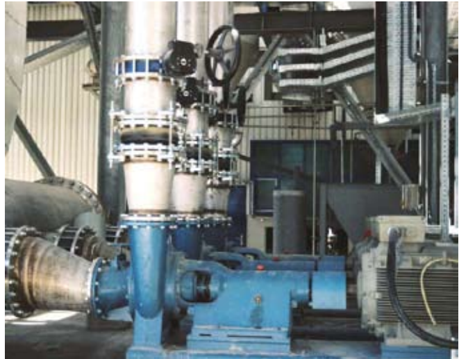
Center Line ® RS installed in a juice purification system
